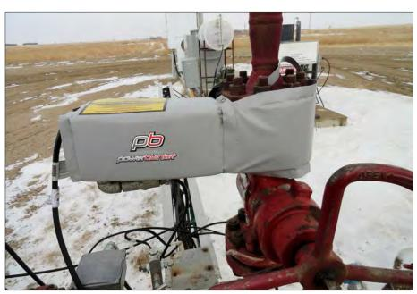
On-site Valve & Instrumentation Heater
