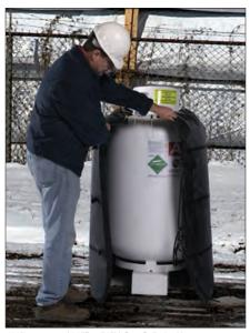
420lb propane / 30"D x 52"H Gas Cylinder Heater
