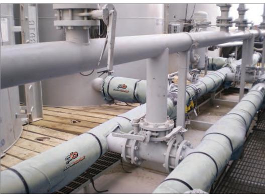
On-site Pipe & Manifold Heating System
